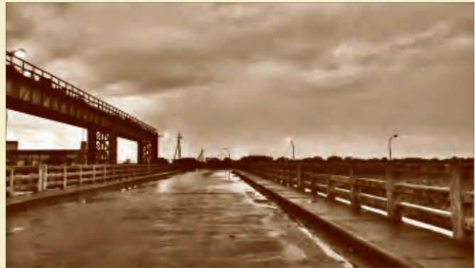
Mahanadi Barrage Cuttack
