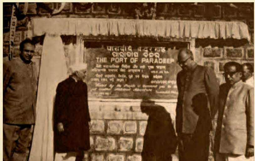
On 3 rd January 1962, the foundation stone of the Paradeep Port was laid by Pandit Jawahar Lal Nehru in the presence of Shri Biju Patnaik
