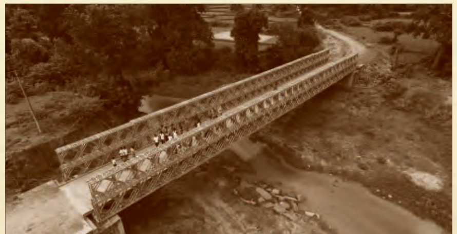
Steel Bailey Bridge
