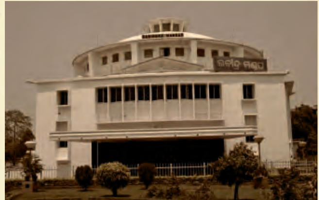
Renovated Building of Rabindra Mandap at Bhubaneswar
