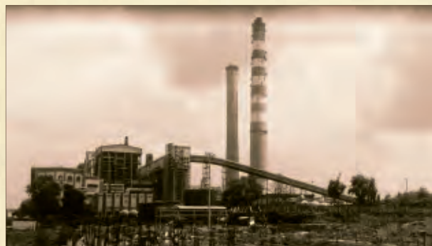
IB-Thermal Electrical Project at Banharpali, Jharsuguda
