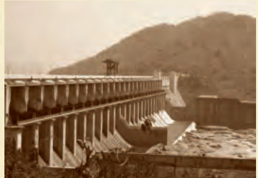
Rengali Hydro-Electric Project
