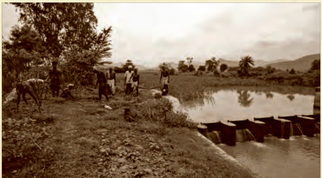
Check Dam constructed under the Mukhya Mantri Adibandha Tiyari Yojana (MATY)
